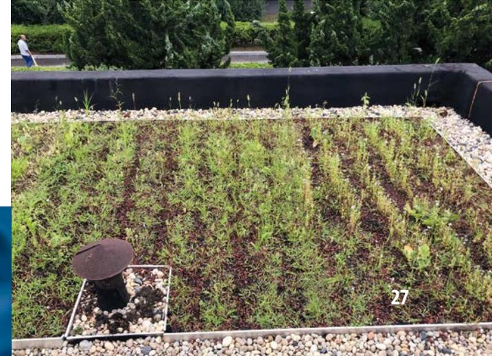
In this pilot project the following parts of the HWT-system were applied: SkinRoofing, in three different sections mentioned before, HWT-drainy rain pipe, and a green wall, supplied by Sempergreen. The eventually overflowing water irrigates the surrounding garden with orchards and viticulture. The whole system is equipped with measuring instruments, which can be supervised in the Netherlands via Wifi. The project opened at the first of June 2017 with a festive seminar.
